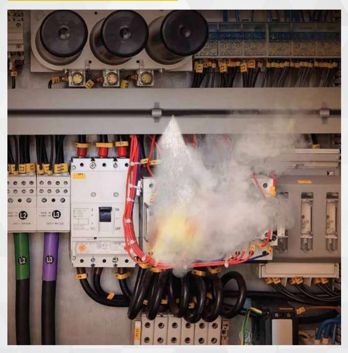
IN-PANEL TUBE BASED MICRO-ENVIRONMENT SUPPRESSION SYSTEM (CQRS)
